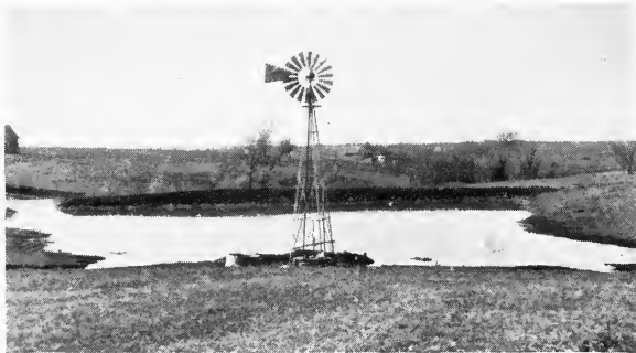
Figure 42.—Small Missouri individual-farm reservoir with earth dam.
